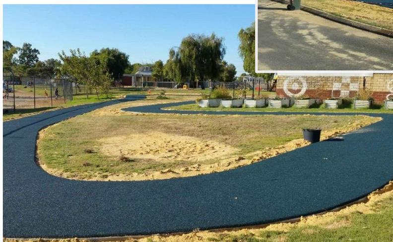
The 20mm of rubberised softfall has now been laid. Next step is to mark up the track with lines which is planned for this coming weekend.
